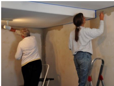
Nancy Miehle and Tami Roleff painting along the ceiling
