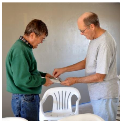
Bob Miehle & Jim Melchert preparing to install the new hanging system
